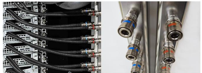
Since the manifolds occupy additional space in the rear of the rack, a DLC rack is usually deeper than an air-cooled rack. The typical depth of a DLC rack is 1,400 mm.
